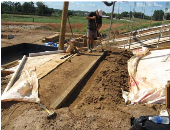
Figure 1. Installing Wattle on Curb with "tail" in 4-inch Trench; Backfilled with 2 inches of Soil
