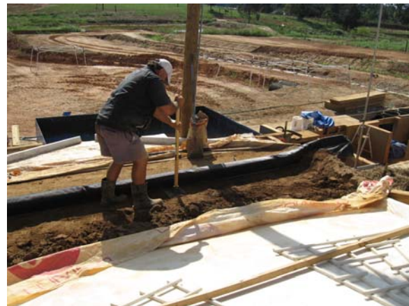
Figure 1. Installing Wattle on Curb with "tail" in 4-inch Trench; Backfilled with 2 inches of Soil
